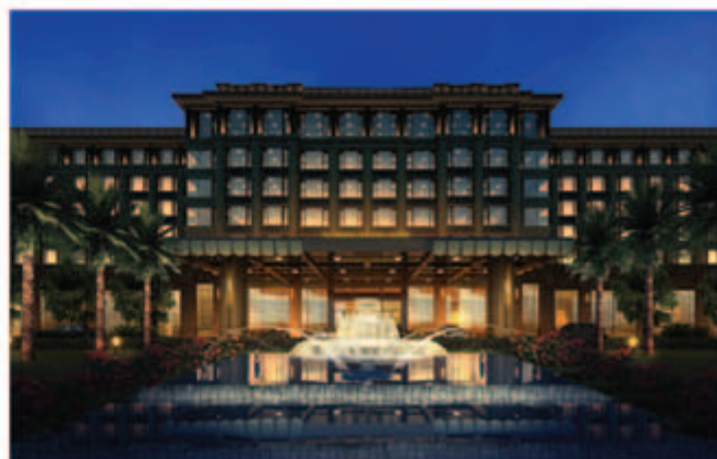
■ Regal Yuhong Hotel (2016) - Zhengzhou, Mainland China (*)
