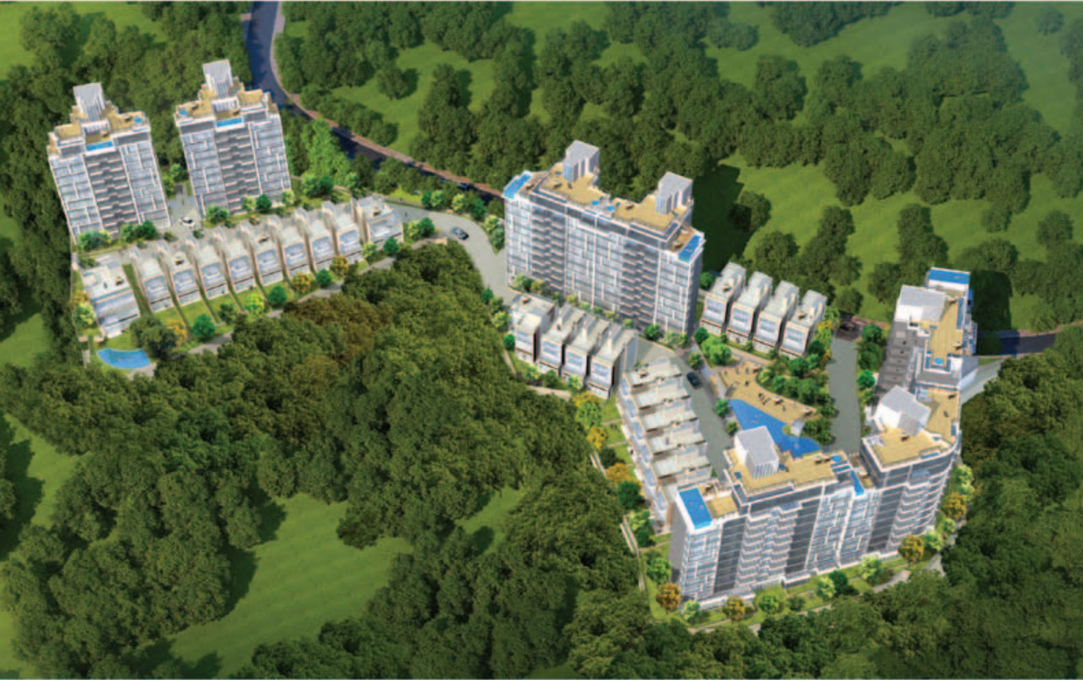
■ Luxurious residential development at Sha Tin Town Lot No. 578, Area 56A, Kau To, Sha Tin, New Territories - foundation works in progress (*)
