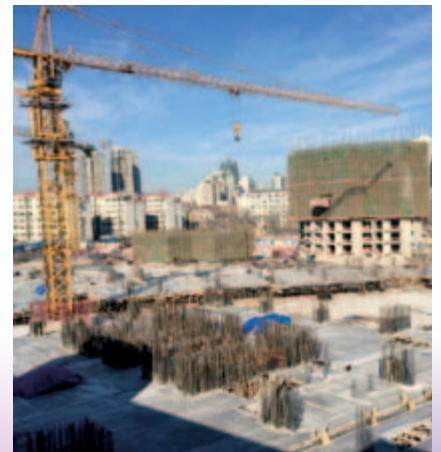
■ Superstructure works of the residential towers of the composite development in progress
