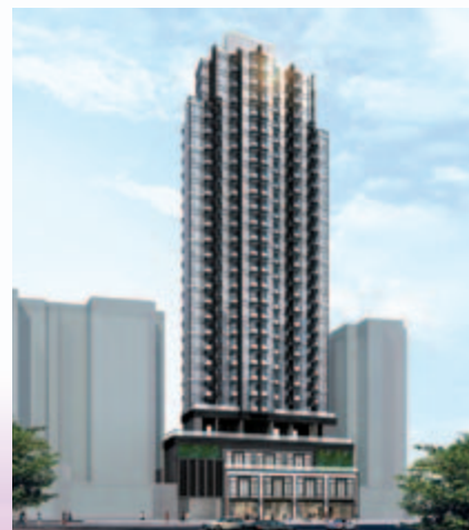
■ Commercial/residential development at Nos. 69-83 Shun Ning Road, Sham Shui Po, Kowloon – superstructure works in progress (*)
