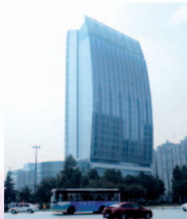
■ Regal Xindu Hotel, a five-star hotel in the first stage of the composite development – superstructure works completed
