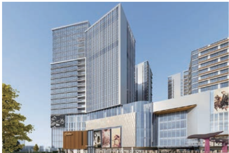
Commercial/office towers of Regal Cosmopolitan City (*)
