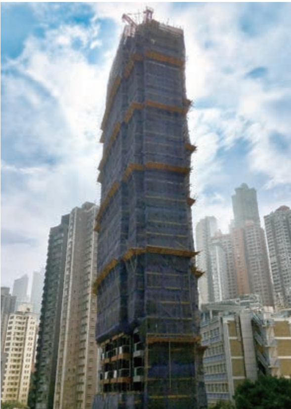
Superstructure works in progress
