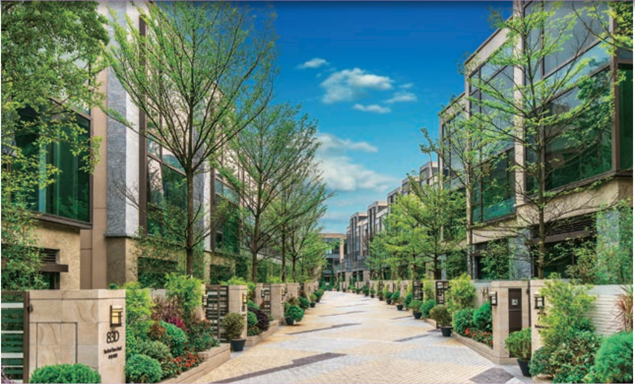
Casa Regalia, the garden houses in the residential development at Nos. 65-89 Tan Kwai Tsuen Road, Yuen Long, New Territories
