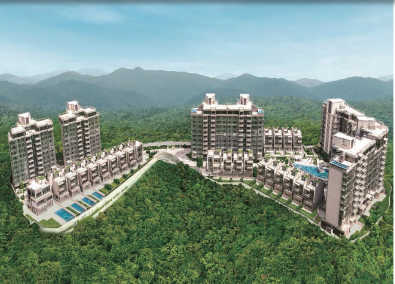
Mount Regalia, a luxurious residential development at 23 Lai Ping Road, Kau To, Sha Tin, New Territories
