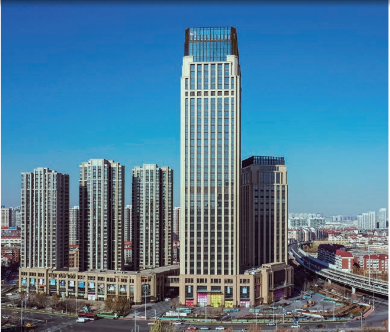
Regal Renaissance, a composite commercial/office/residential development in a prime location of Hedong District, Tianjin
