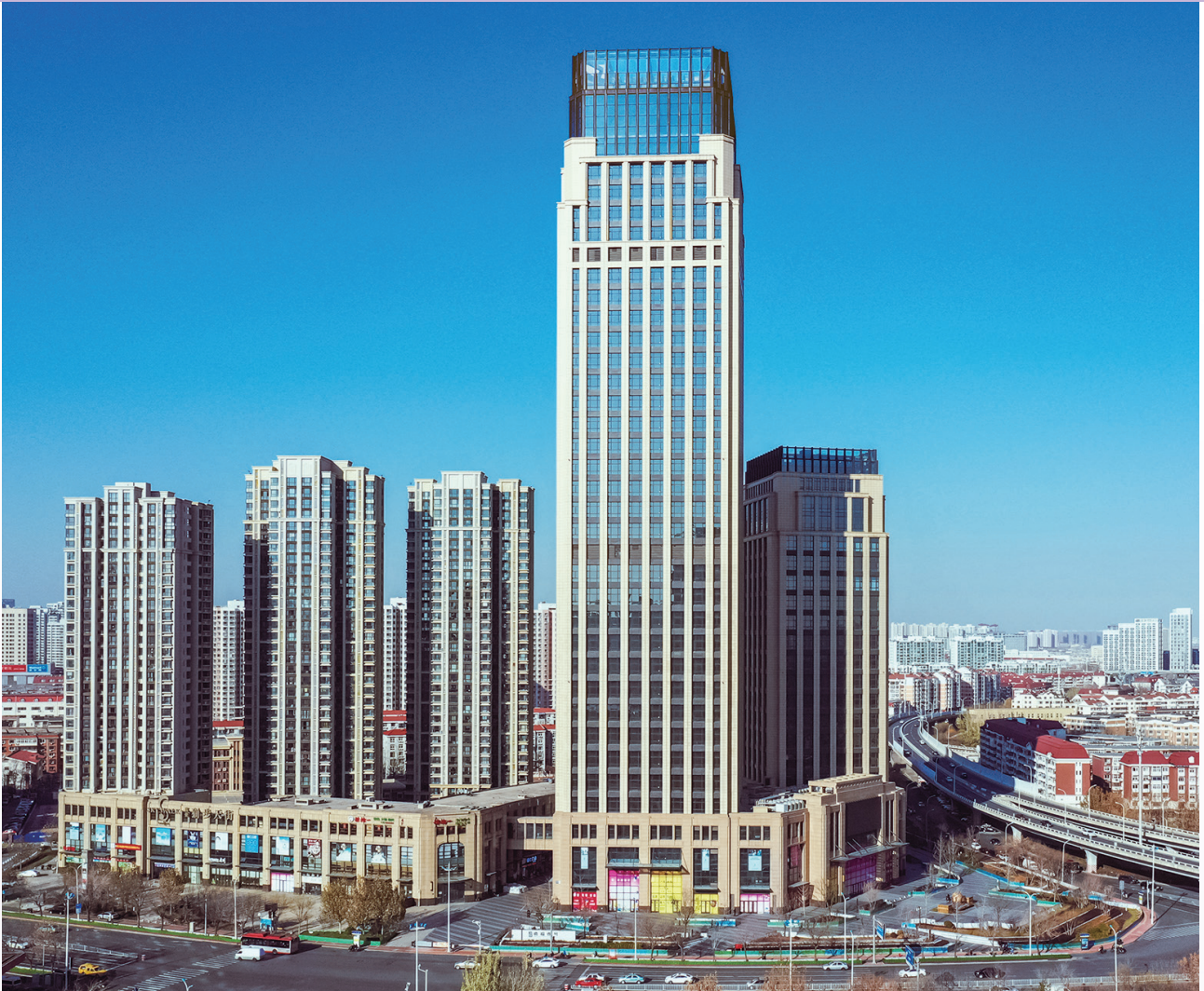
Regal Renaissance, a composite commercial/office/residential development in a prime location of Hedong District, Tianjin
