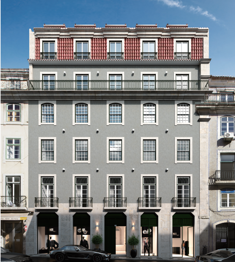
Fabrik, Rua Dos Fanqueiros 156, Lisbon, Portugal (*) - rehabilitation renovation works completed
